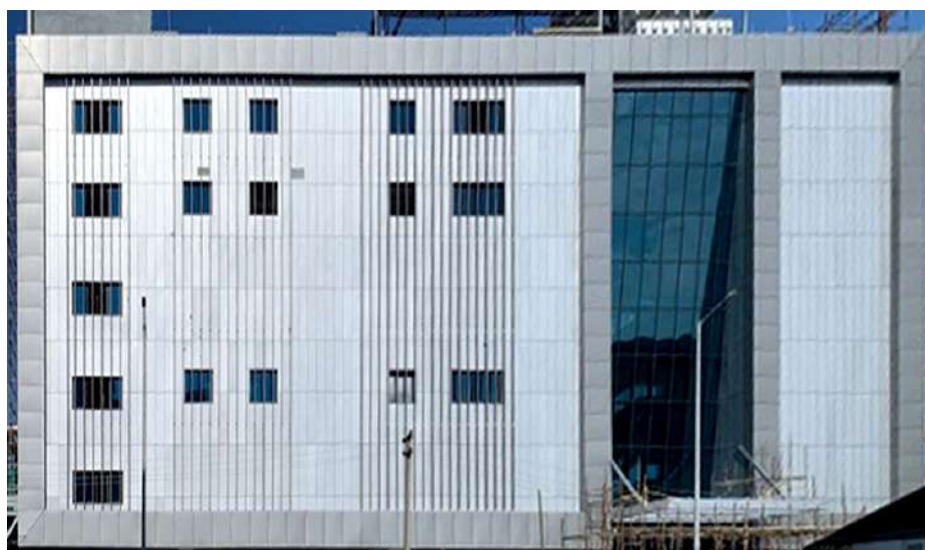
▼ Fig 1.7 : National Data Centre, North East Region
